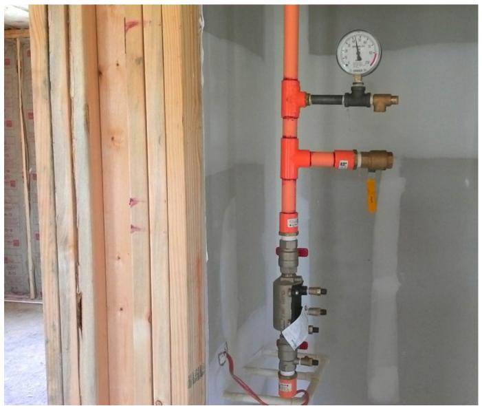
Inspection photos of an NFPA 13D sprinkler system installed in a Homestead at Hartness home. The sprinkler systems cost about \$2,000 per unit installed, or about 1 percent of the per-unit cost of roughly \$208,000. Photographs: Jeff Nelson, fire marshal, Boiling Springs Fire Department
